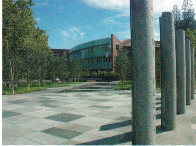
The plaza itself is paved in a combination of the stones used for other components of the project – Prairie Green, Abyss Green and Peribonka – all done in a thermal finish. (Photo courtesy City of Walnut Creek, Calif.)
