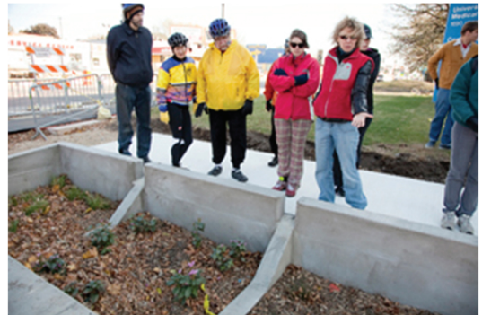
Christine Baeumler, an art professor at the University of Minnesota, described the function and structure of a "tree trench" and storm water planters that will be built into the Central Corridor light rail project. (Photo: Matt M. Johnson)
