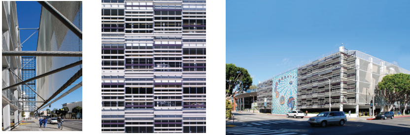
Left to right: Gehry's mesh screen still remains on one surface; panels are made of colored cement board; a colorful tile mural by Anne Marie Karlsen adorns one facade (Ball-Nogues created another art piece).
