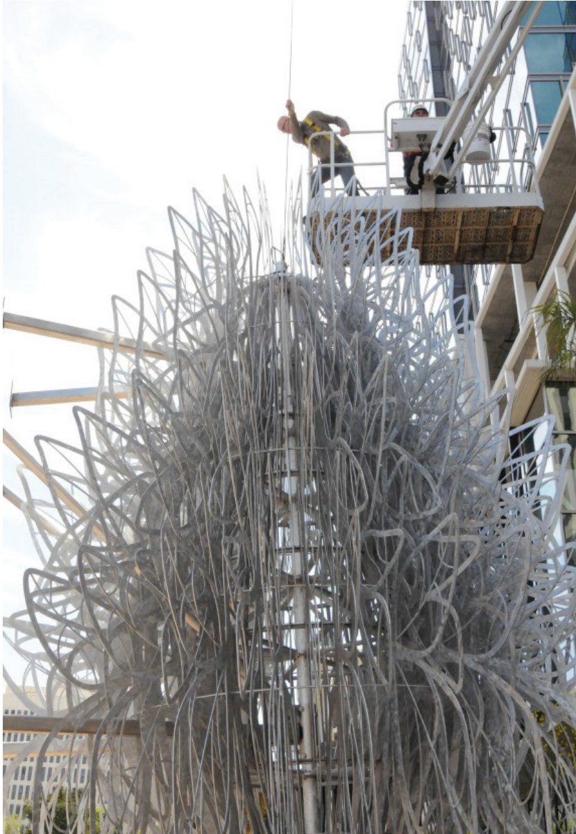
Cliff Garten oversees installation of his Lotus-inspired art piece.
